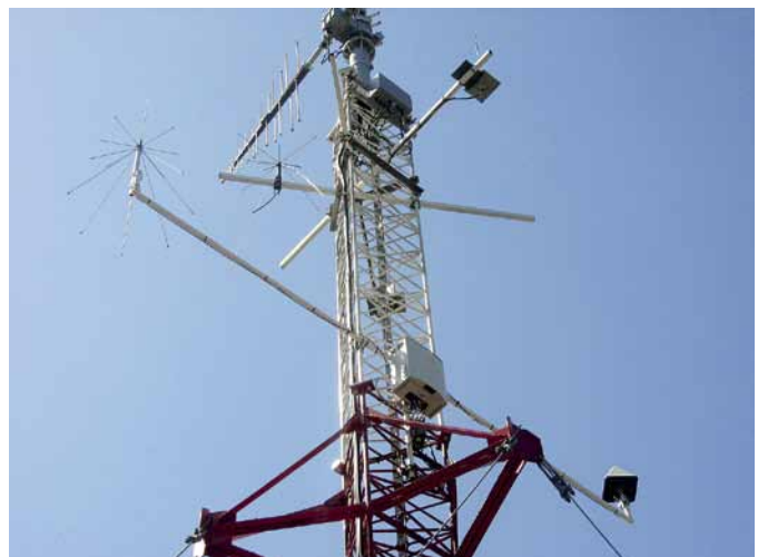
FIG 1 R&S®UMS 100 monitoring systems integrated into main stations are mounted on the common antenna mast below the DF and monitoring antennas and the rotor.
